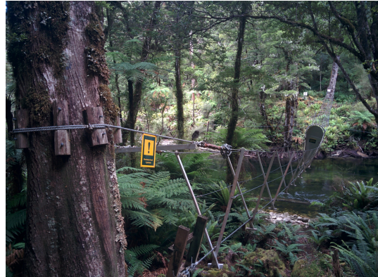
A bridge with low capacity
